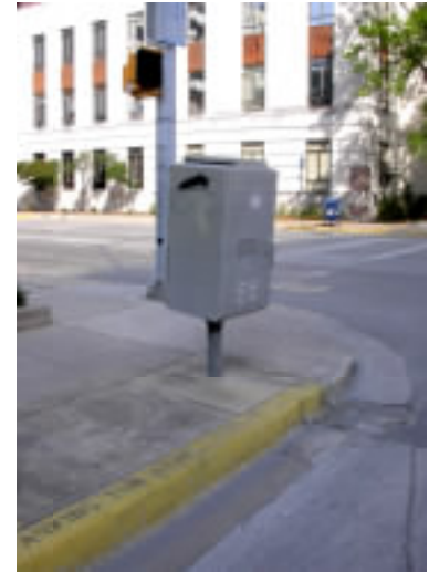
a utility box blocking a busy sidewalk creates a conflict with pedestrians
