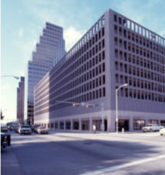
an example of a garage that includes pedestrian spaces at the ground level
