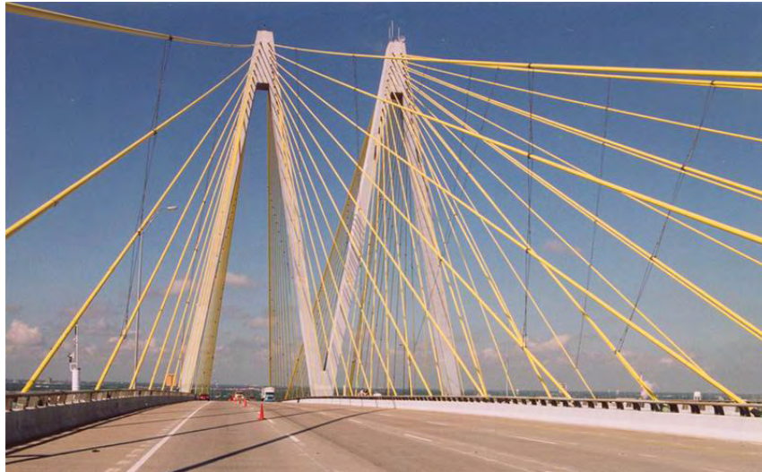
Figure 6.26 Cable networks formed with cross-ties
