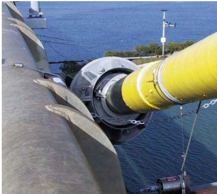
Figure 6.22 Freyssinet damper installed on stay AS24
