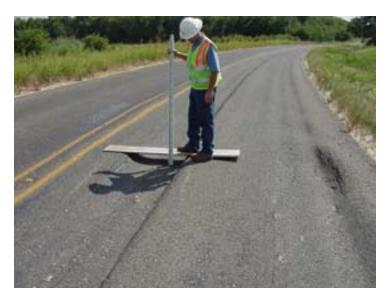
Figure 3.2 Example of Damage Done by Grain Haulers (Source: Mike Murphy, 2003)
