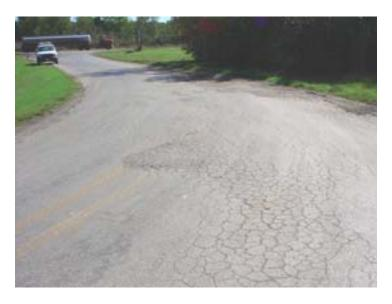
Figure 3.4 Example of Damage Done by Oil Field Trucks (Source: Mike Murphy, 2003)
