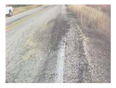
Figure 3.5 Example of Damage Done by Salt Water Trucks (Source: Mike Murphy, 2003)
