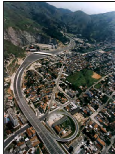
Figure 2.15 South African toll road
