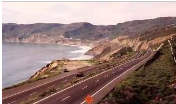
Figure 2.14 Mexican toll road
