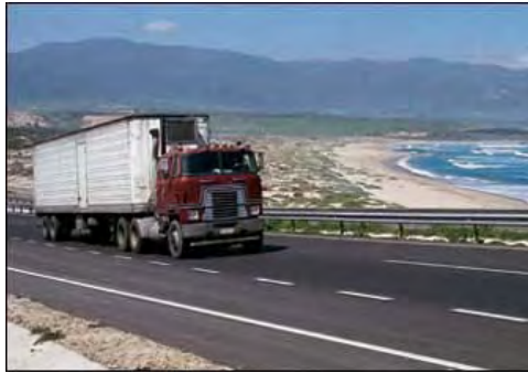
Ruta 5 Toll Road, Chile
