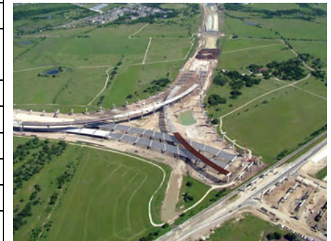
SH 130, under construction, Central Texas
