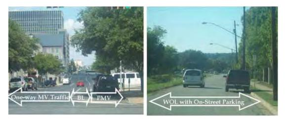
Figure 3.4: Examples of one-way streets with BL (left) and WOL (right) and motor vehicle parking on-street
