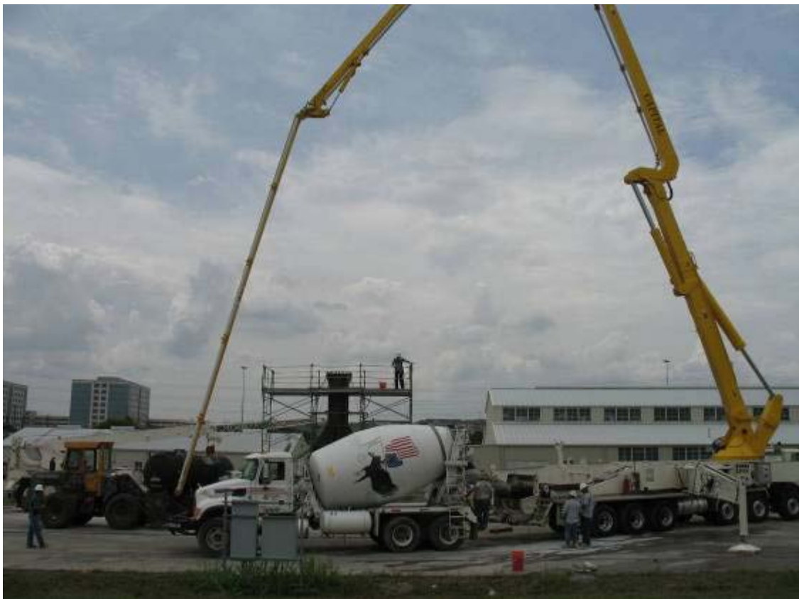
Figure 2.2.13 - Priming of concrete pump.
