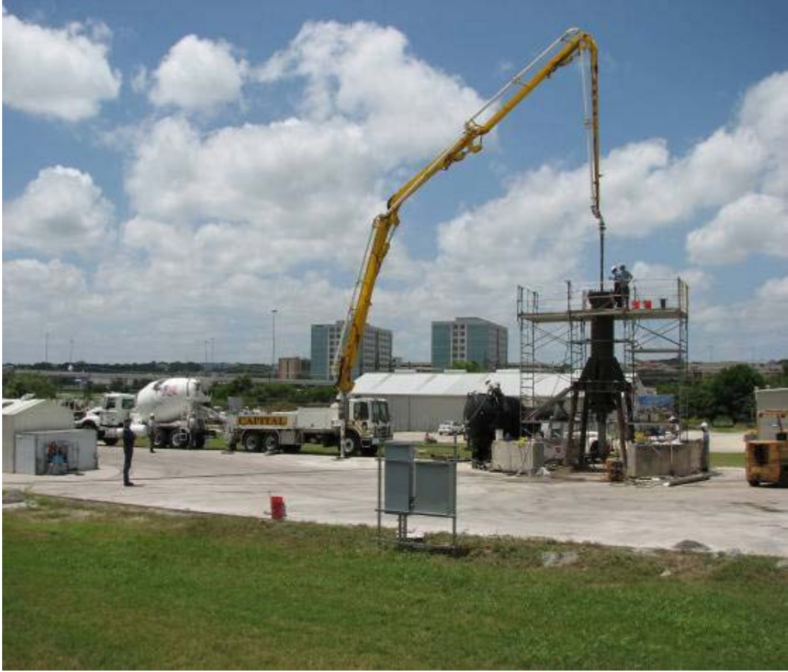
Figure 2.2.17 Complete Setup. Date: 08/07/2007, Ht of Drop: 70'
