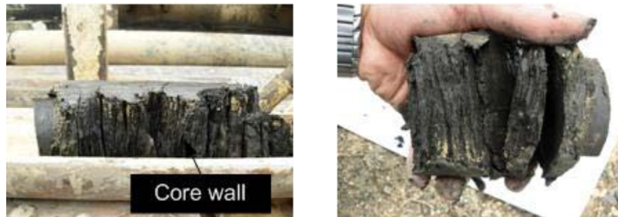
Figure 1.6.8 Extruded sample from the side wall of the verification core (#5)
