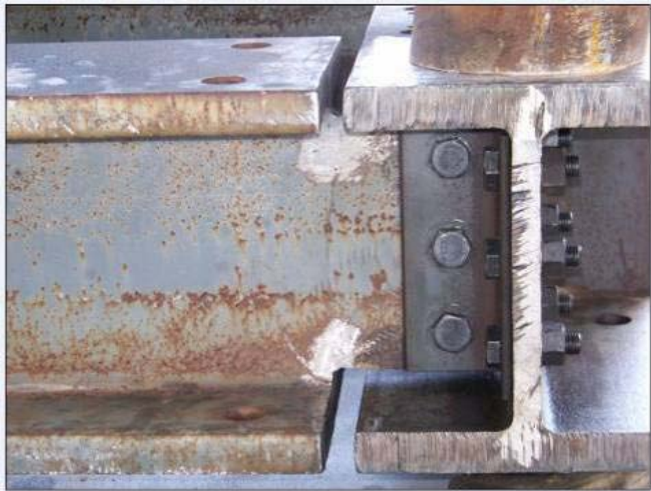
Figure 2.3.18 - Double angle shear connection between beams
