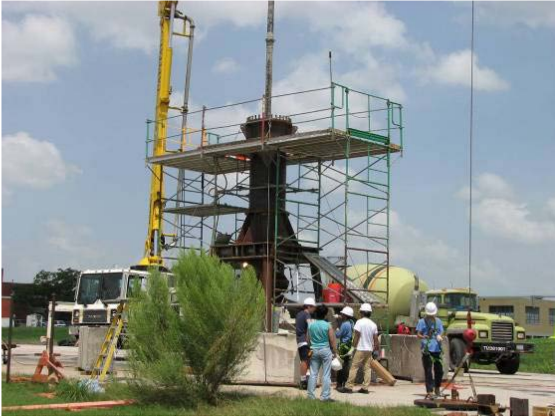
Figure 2.2.15 Complete Setup. Date: 07/30/2007, Ht of Drop: 30'
