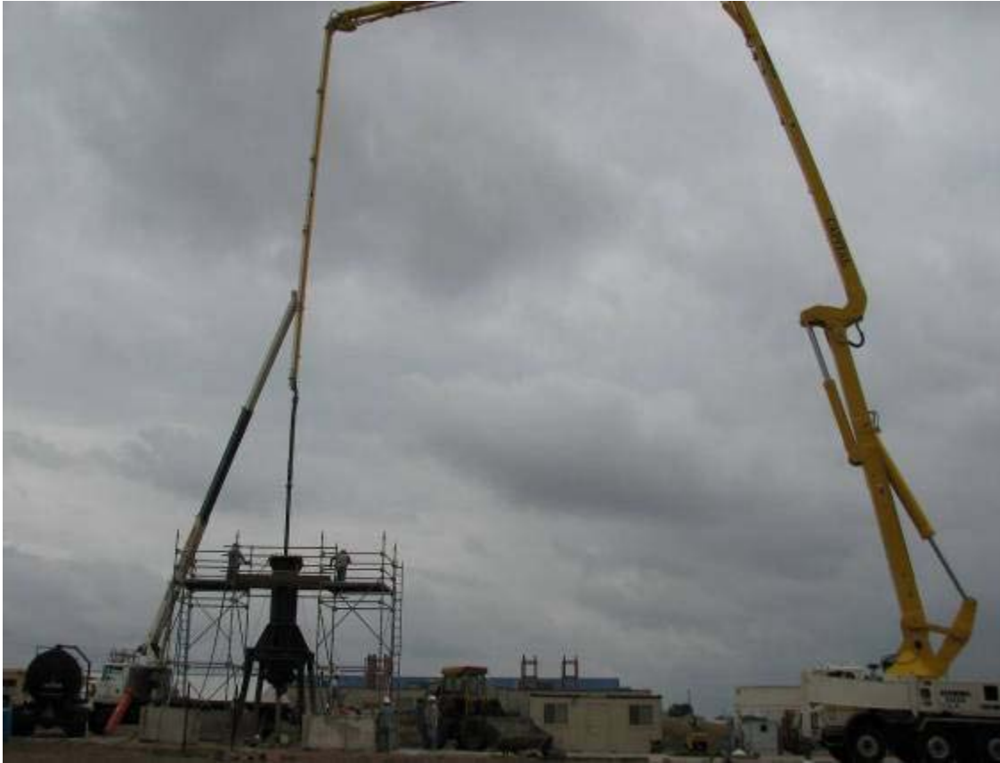
Figure 2.2.18 Complete Setup Date: 02/15/2008, Ht of Drop: 100'
