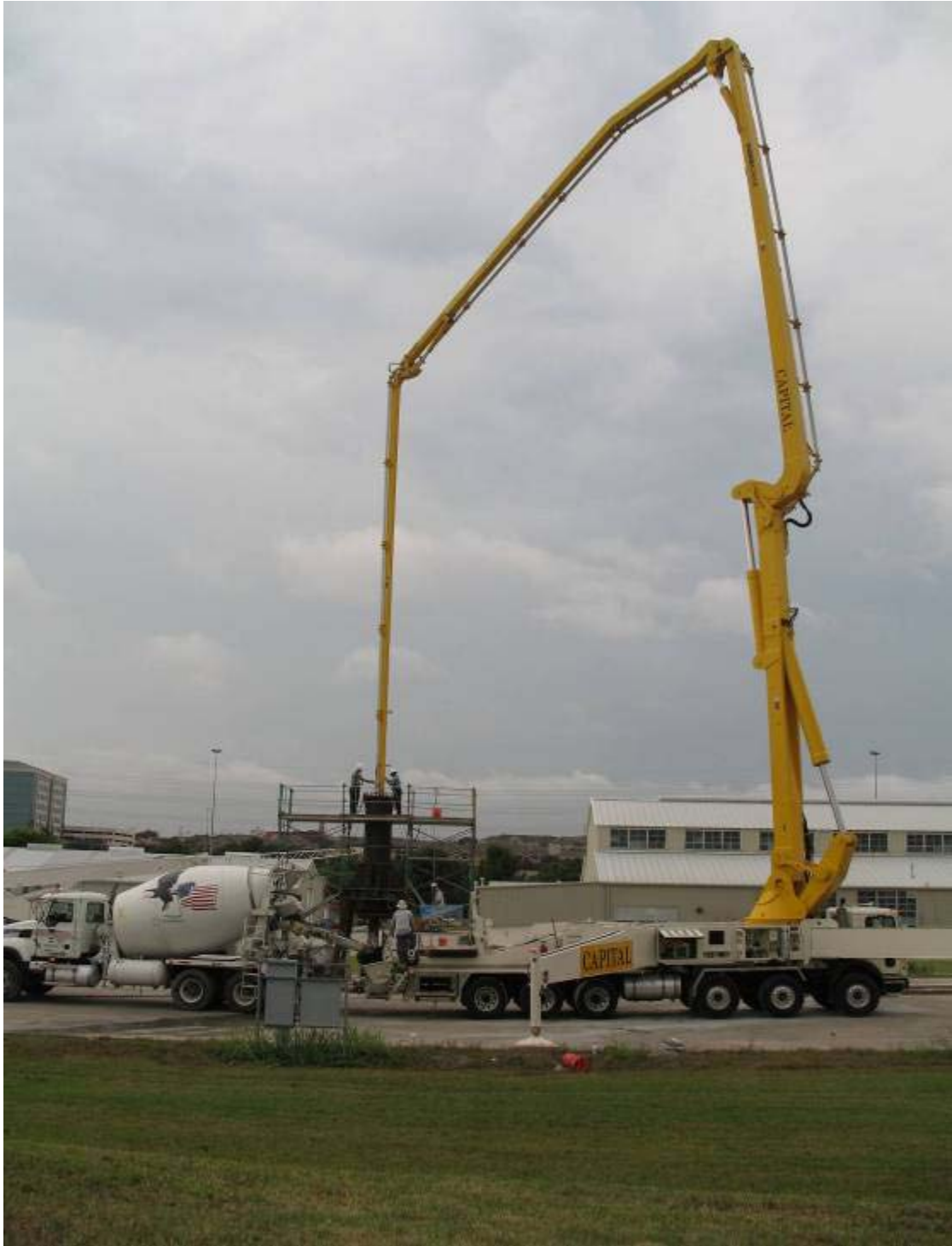
Figure 2.2.16 Complete Setup Date: 08/01/2007, Ht of Drop: 70'
