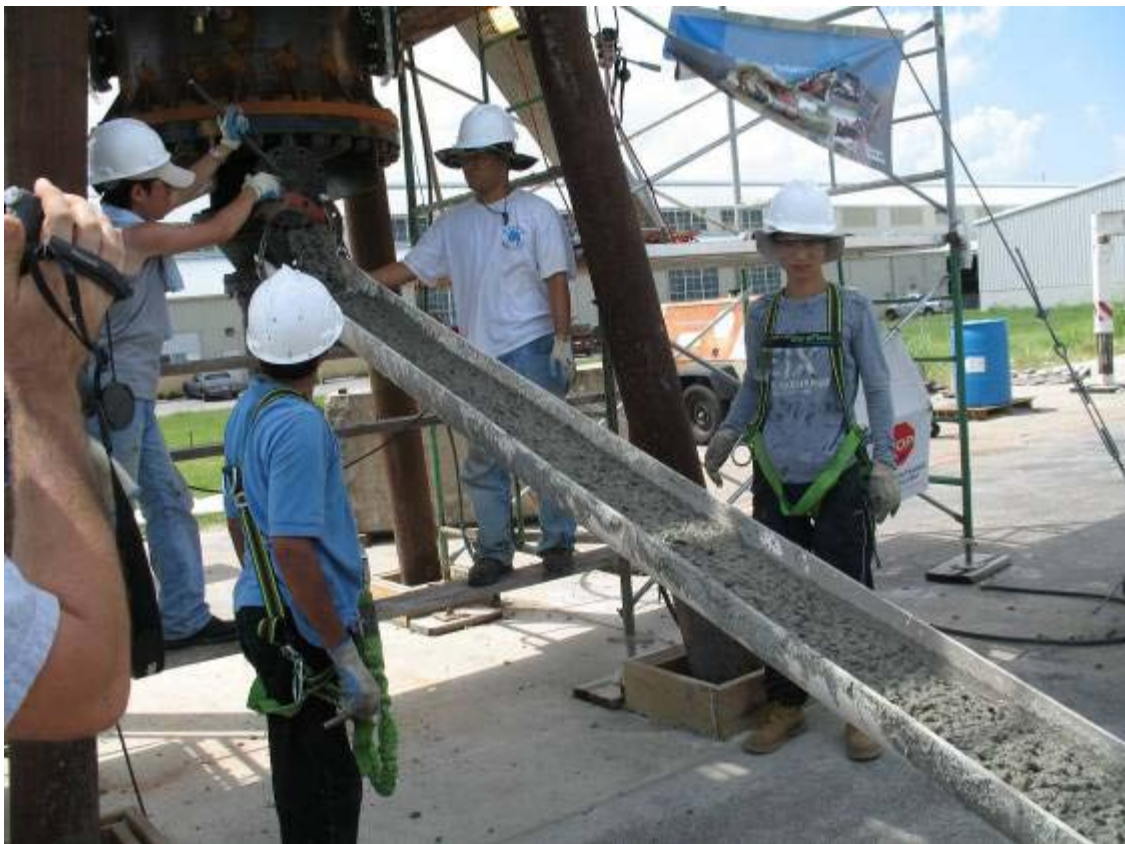
Figure 2.2.14 – Evacuation of concrete from the rocket
