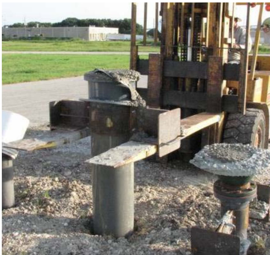
Figure 2.2.22 – Placement of PVC pipes
