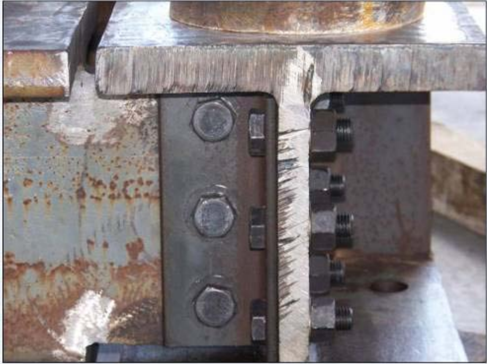
Figure 2.3.17 – Double angle shear connection between beams
