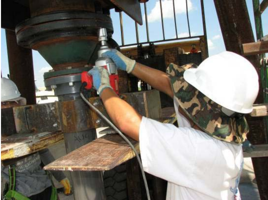
Figure 2.2.10– 6” Clear PVC pipe attached through a reducer
