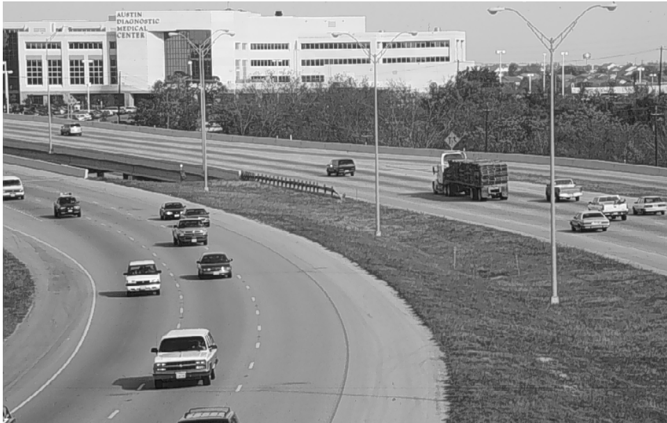
Figure 2.1 MoPac at Walnut Creek Filter Strip
