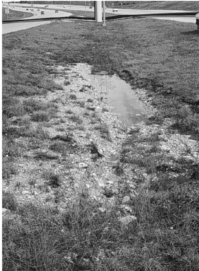
Figure 2.4 Erosion at the Walnut Creek Vegetated Buffer Strip
