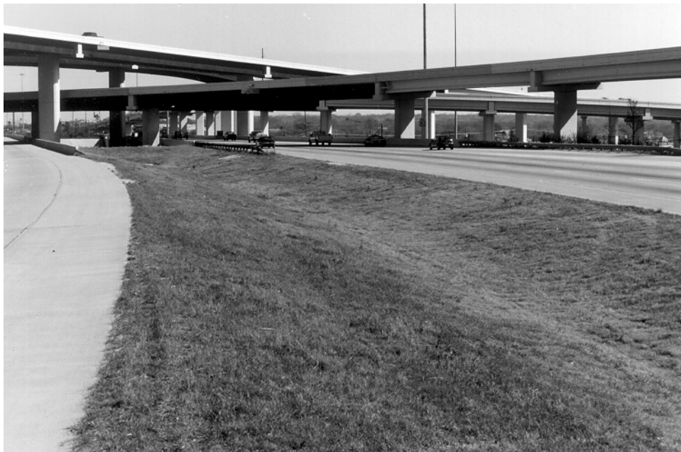
Figure 2.2 Vegetated Buffer Strip at US 183 Site
