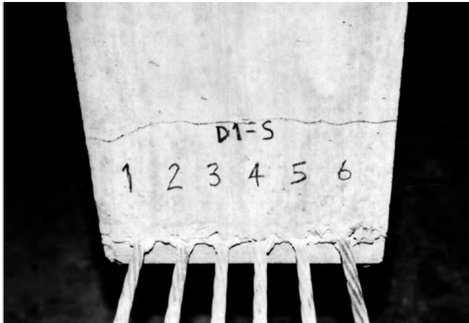
Figure 3.4 Tensile crack at beam end
