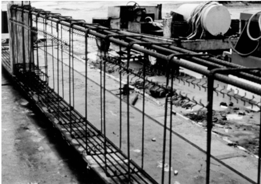
Figure 3.2 Mild steel reinforcement
