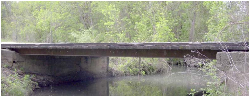
Figure 1.1 Bridge at County Road 108 and Boggy Creek
