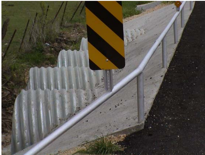
Figure 1.6 New Guard Rail Installed at Culvert
