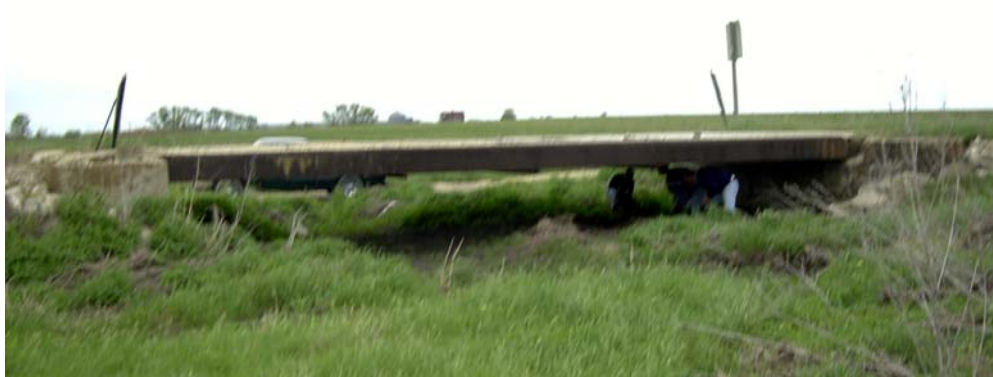
Figure 1.2 Bridge at County Road 230 and Boggy Creek
