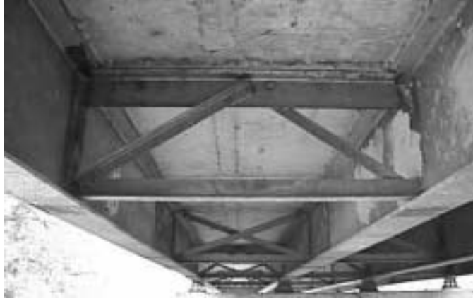
Figure 1.10: K-type and X-type diaphragms
