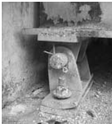
Figure 1.3: A rocker support at an abutment
