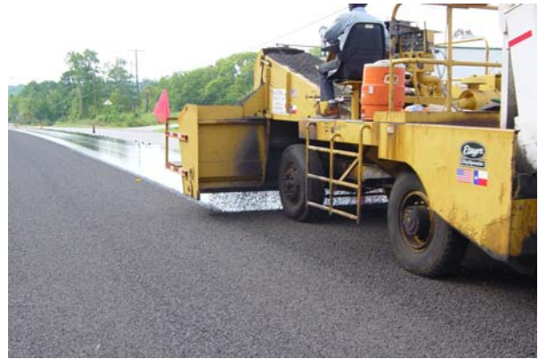
Seal Coats for Pavement Preservation by Tom O'Leary, Ergon Asphalt & Emulsion
