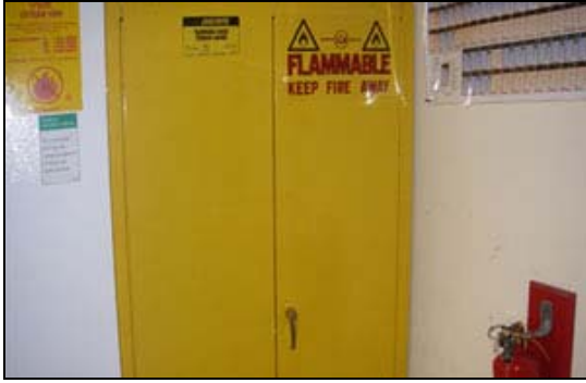
Proper storage of flammable chemicals
