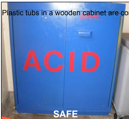
Proper acid storage
