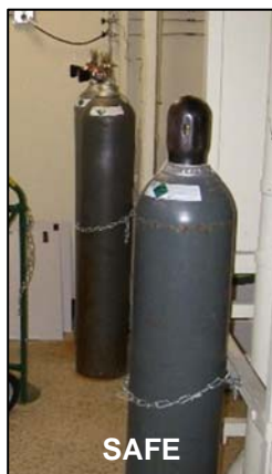
Acceptable method of securing a gas cylinder
