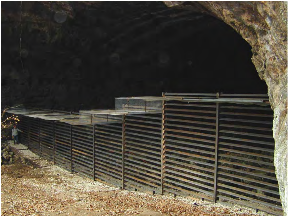
The world's second largest cave gate, Great Spirit Cave, Pulaski County, Missouri. The half gate weighs 18 tons and is 101 ft. wide and up to 14 ft. tall. Completed in October 2002, it protects endangered Gray and Indiana bats and multiple resources. By Mike Slay.
