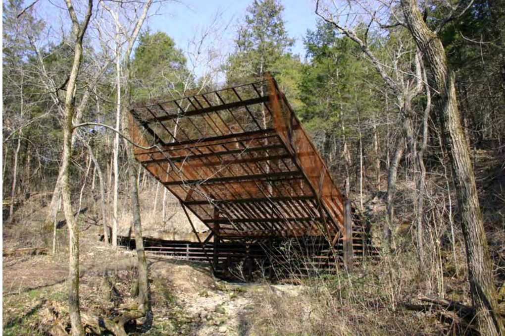
The “chute gate” at Tumbling Creek Cave, Taney County, Missouri. The rectangular, expanded-metal chute allows maternal Gray bats to access the cave. The colony increased after the gate was built, April 2004. By Bill Elliott.
